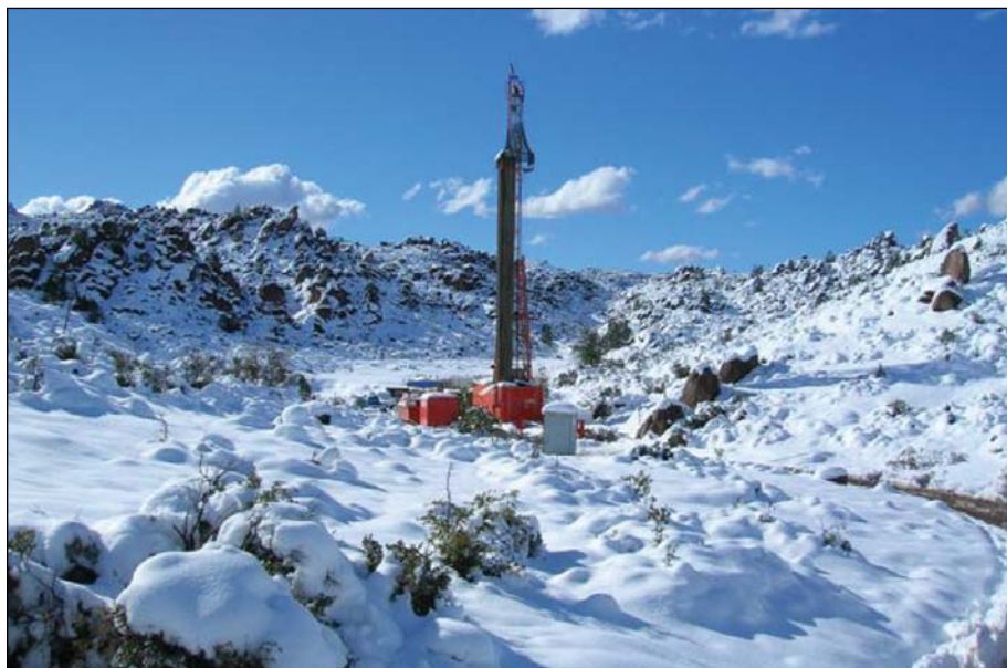
This Chicago Pneumatic CP50 rig was working through winter in the US (Fig. 2; photo by Dennis McLeod, provided by Major Drilling Group International Inc.).
